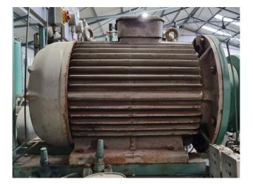
ofgor nl® ASYNCHR.MOT3~TYPE XKE250M02 60 3/85 No 7044835 PSS kW S1 50 Hz V 400 98A COS 9 2970min -Isol. 457 kg .10411
